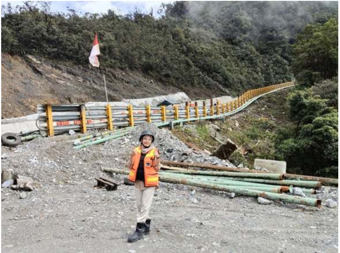
Inspeksi area MSR ( Mine Supply Road )
